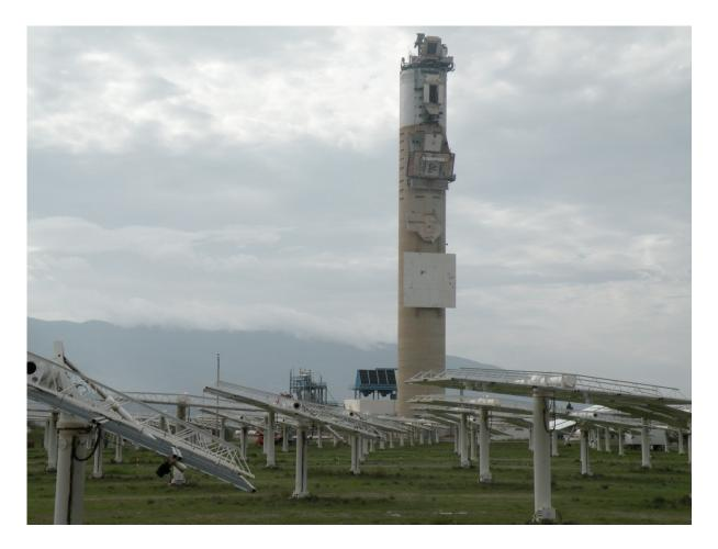
This is a Solar Tower Power Plant CESA-1, with 300 heliostats with 40 m<sup>2</sup> each, 7 MWth, 83 m height.
